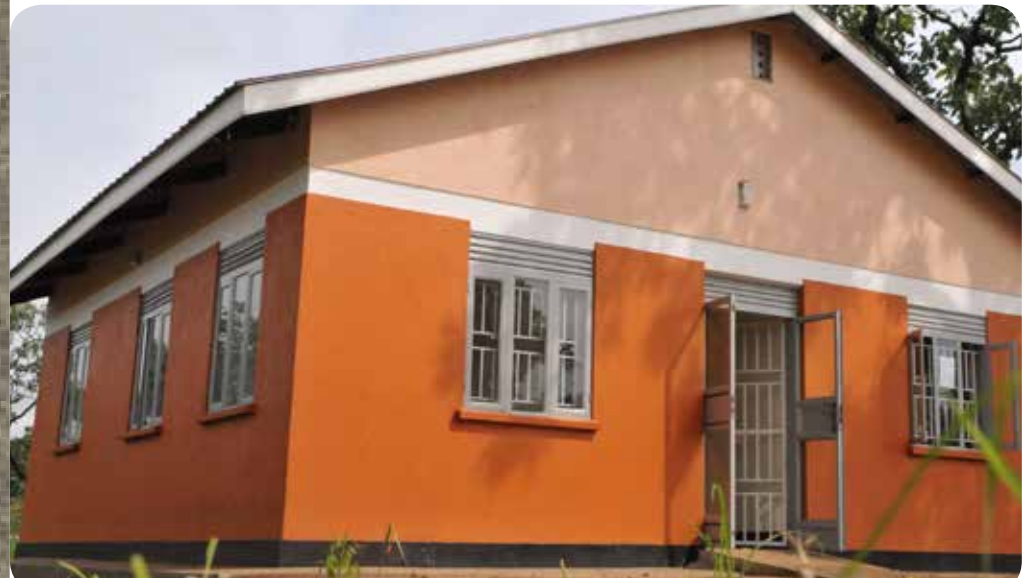
Newly constructed OPM office with solar power installation in Ayilo II A.
