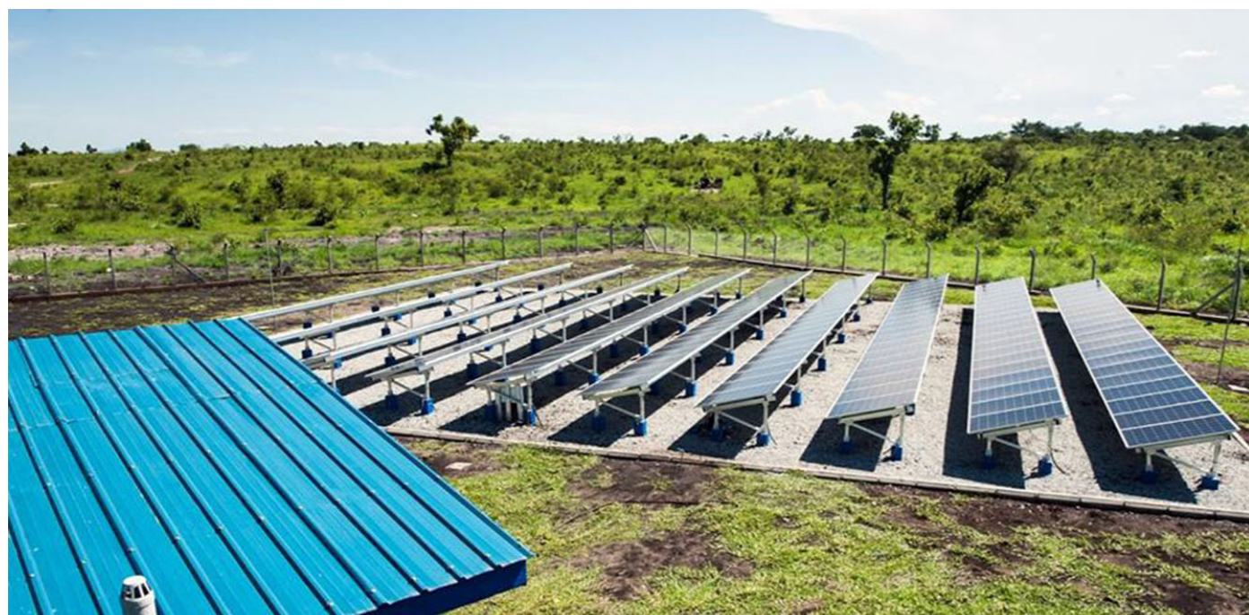
Photo credit: A Solar system that powers a borehole motorized system in Palorinya settlement.
